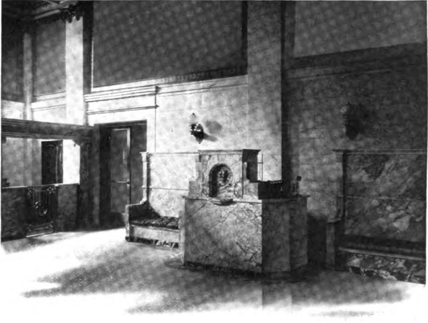
ORNAMENTAL MARBLE DRINKING FOUNTAIN AND SEATS—LOCATED IN THE AMERICAN NATIONAL BANK OF RICHMOND, VIRGINIA. CLEVERLY CONCEALED IN THE SEAT TOPS ARE VENTILATING PIPES FOR ADMITTING PURE FRESH AIR AT ALL TIMES
